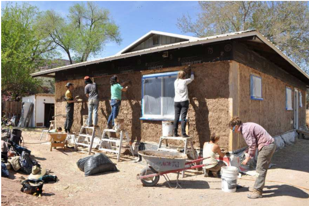
A house made of straw, clay and soil using Permaculture design principles.
